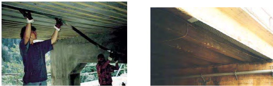
a) Attachment of FRP to the structure b) Final disposition of the FRP
